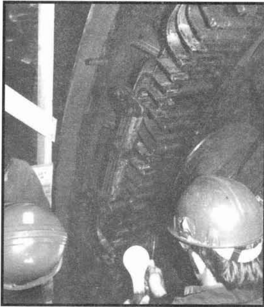
5000 KVA generator undergoing insulation condition assessment after flood.
